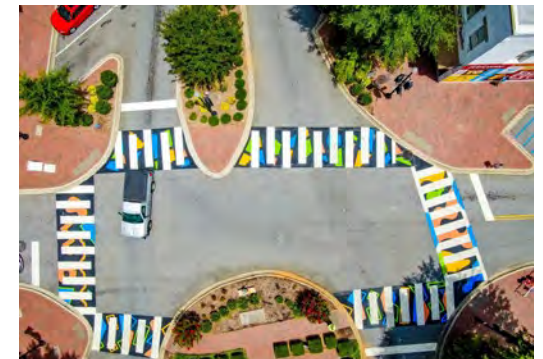
Public Realm Improvements
